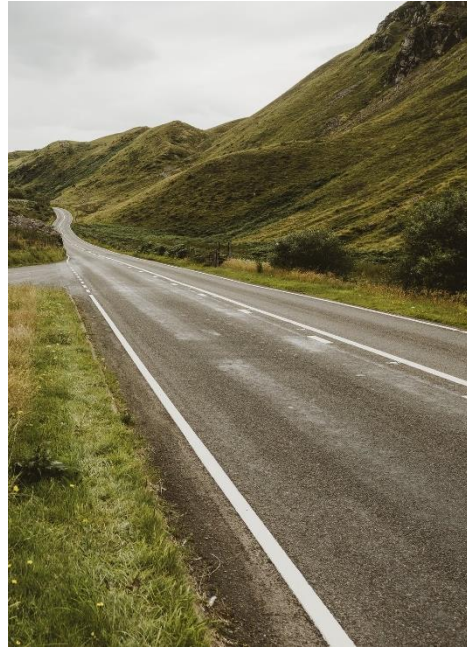
Concrete Road leading the Dam
